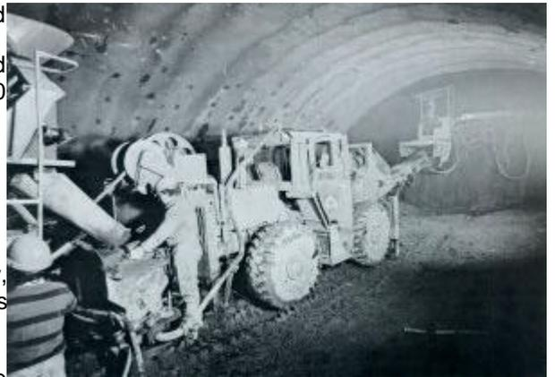
As large tunnels are usually driven from two directions and also in two stages on each side, i.e. roof section and bench section, theoretically four Spray Buffaloes would be needed at a total investment of 3,4 mill. DM.
