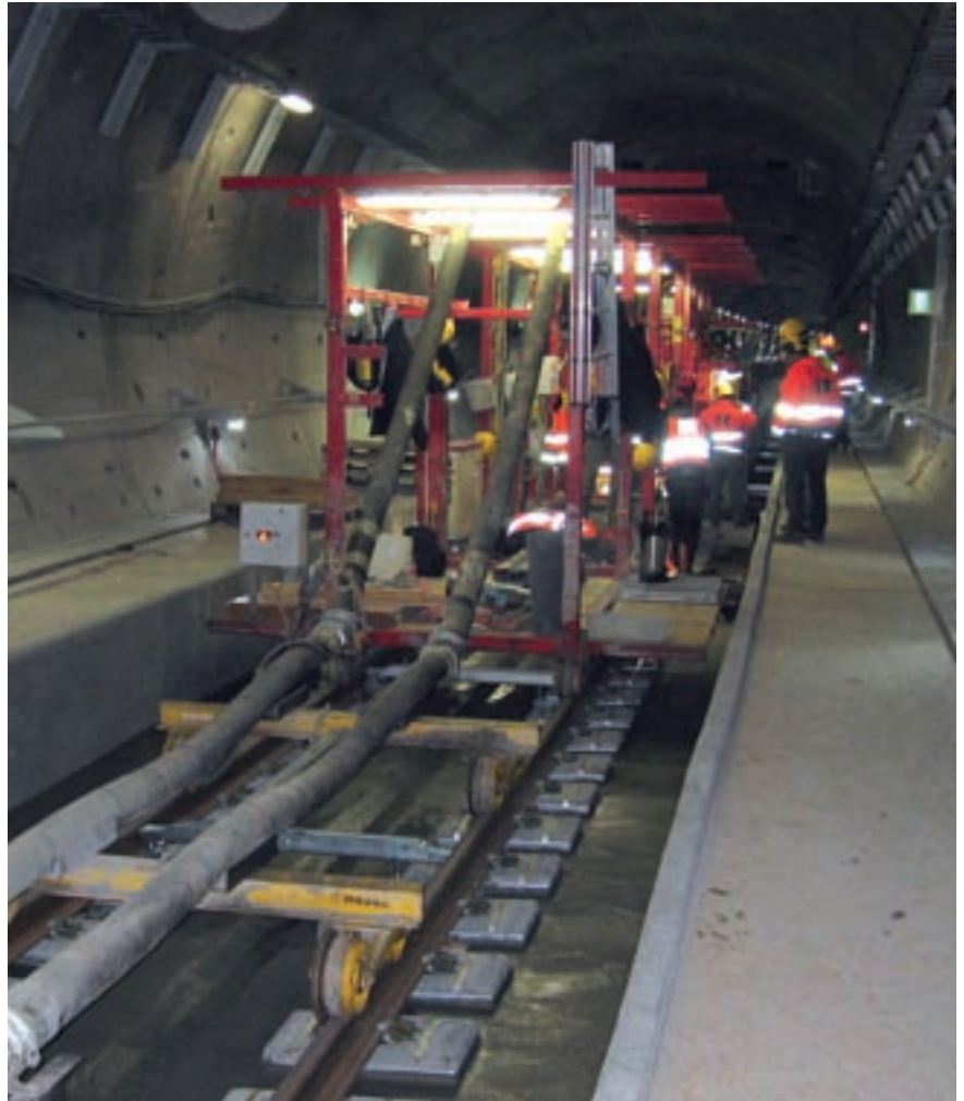
The patented concrete paving machine when embedding the sleeper shoes
