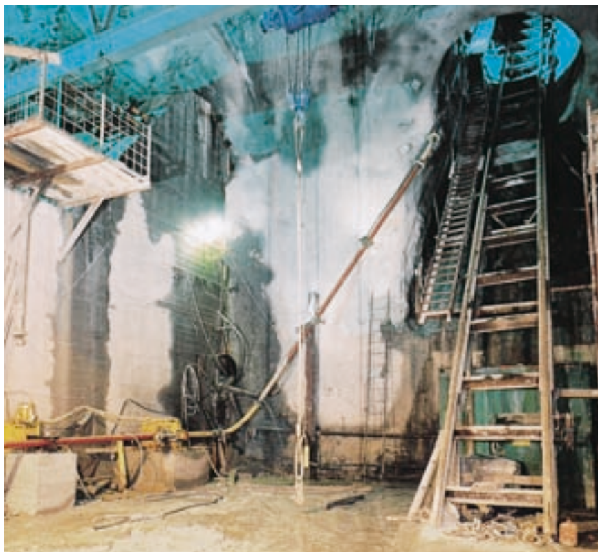
100 mm delivery line with gate valve; to the right, the service tunnel with inclined rail lift
