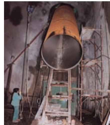
Steel pipe transport through the service tunnel
