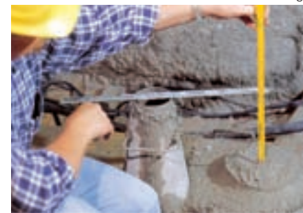
Slump measurement – 22 cm
