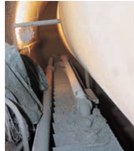
Concrete arriving in the ring space
