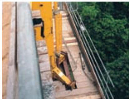
Anchoring of the MXR 24 onto the steel support structure
