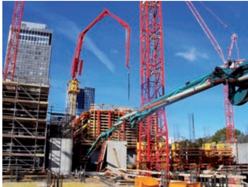
The MX boom stands freely and without ballast on the tubular column, 16 m high
