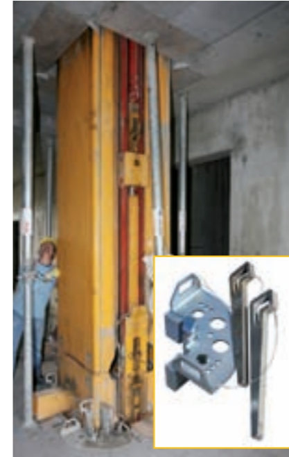
Easy-to-move floor guides keep the boom tubular column laterally fixed
