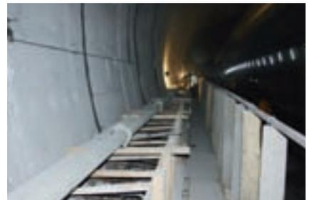
The concrete was pumped over a horizontal range of up to 600 m
