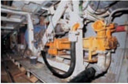
KOV DUO pumps delivered the injection mortar behind the concrete preform
