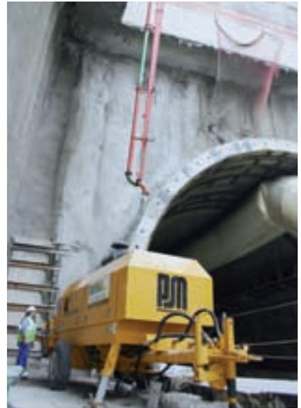
The long-range concrete pumping was performed by a BSA 2109, supplied by a truck-mounted concrete pump situated outside the tunnel
