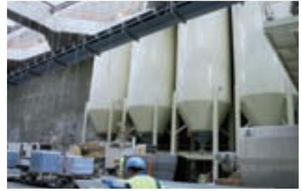
Four KOV 1050s were used to transport the mortar from these reservoirs to the actual injection pumps
