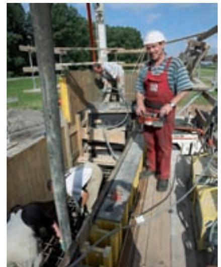
When concreting the narrow reinforcement, the machine operator is as close as possible to the placement site
