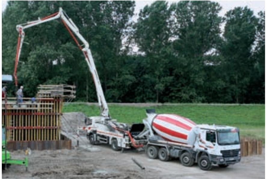
For each bridge section, the BFU concrete pumps have the right boom size. Here is a M 24-4, which will be replaced by two M 52-5 booms in the coming months.
