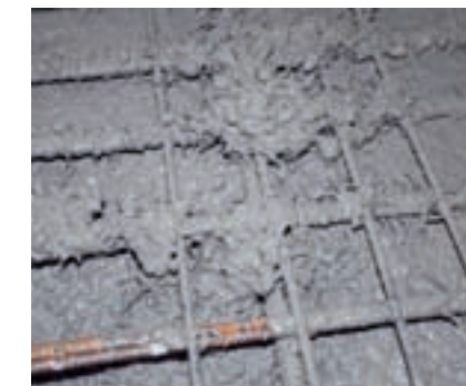
Steel fibre content of 75 kg/m 3 in the concrete
