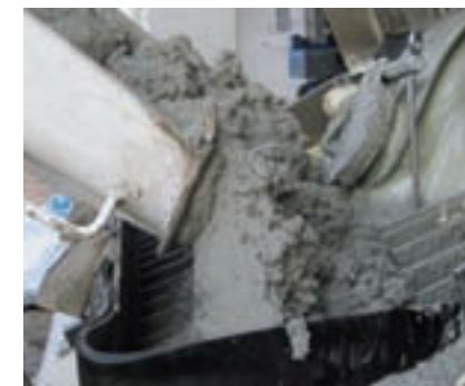
The rigid concrete stands in the hopper
